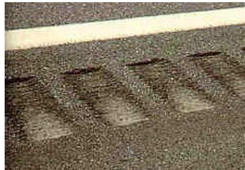
Image is a view of a shoulder rumble strip.
